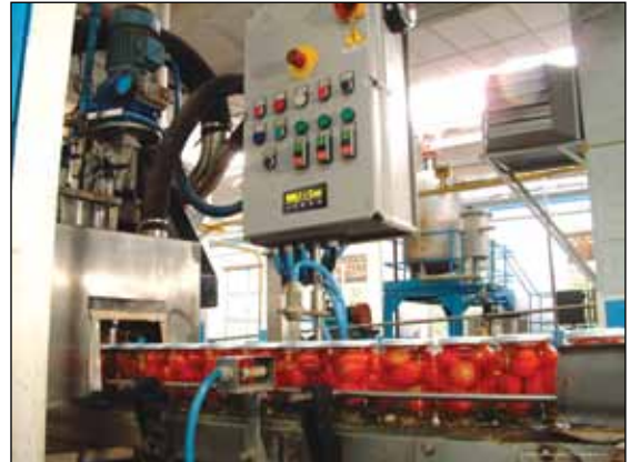
Oven Temperature Monitoring
